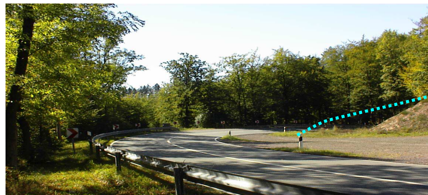
Obstructed view to be cleared
