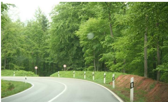
Earth wall instead of guardrails
