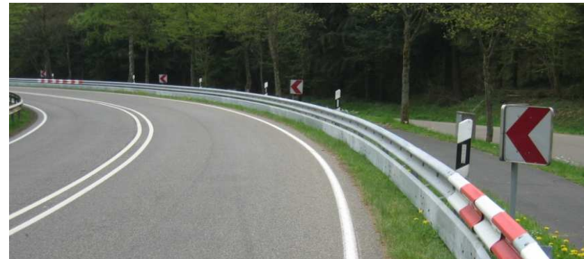
Dispersed signs behind a guardrail
